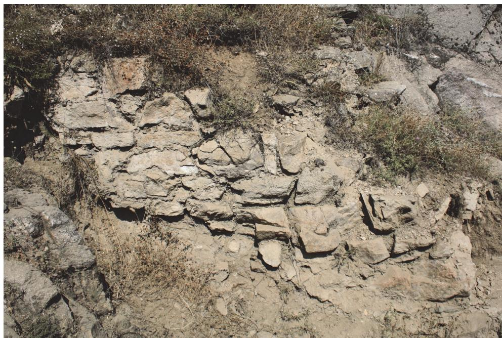
**Fig.6.** Part of the ramparts with emplecton masonry technique, locality "Kitka" - village Bansko (*photography: D.Cvetanov*)
